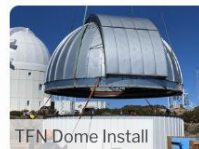
TFN Dome Install
